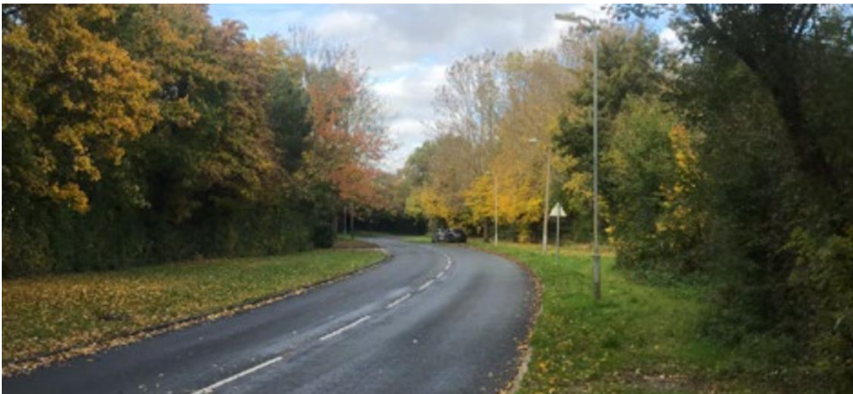
View of site from Far Moor Lane
